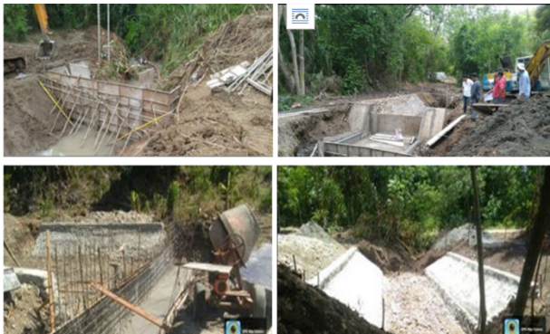
Figure 8: Sediment catchment structures in Diadi, Nueva Vizcaya (top photos) and Cordon, Isabela (bottom photos). Photo Source: NIA-MARIIS
